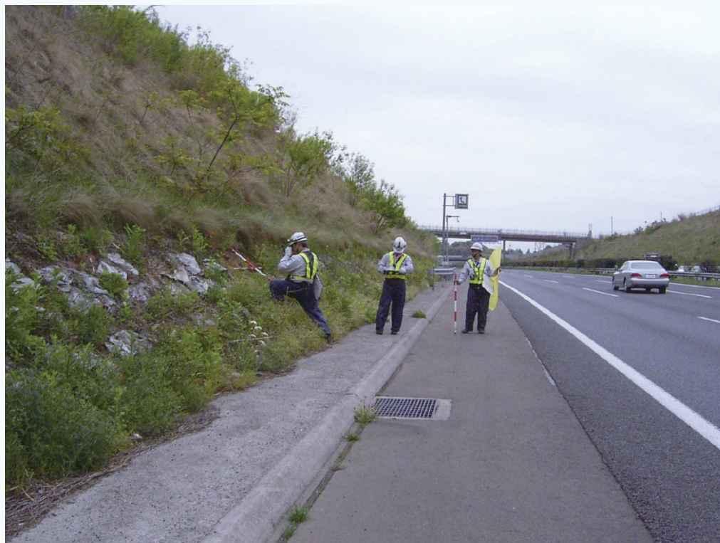
切土のり面の点検
